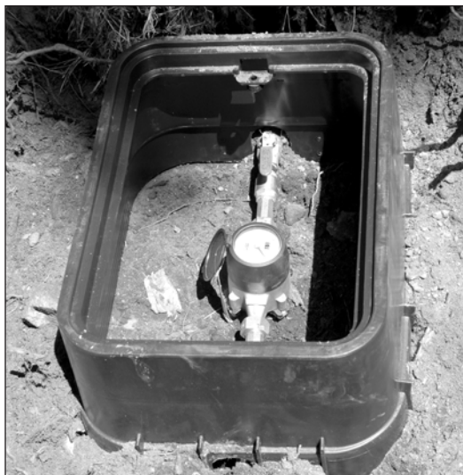
Meter and Low Flow Device Assembly
